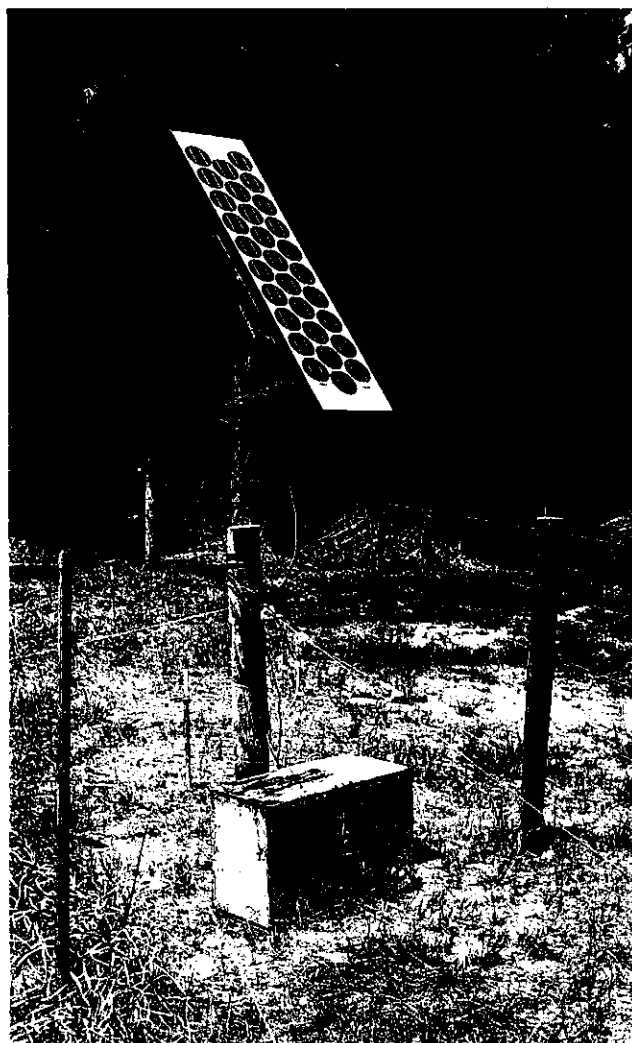
● In remote areas solar energizers power up to 11km of electric fences used for internal and perimeter forest fencing [New Zealand]
